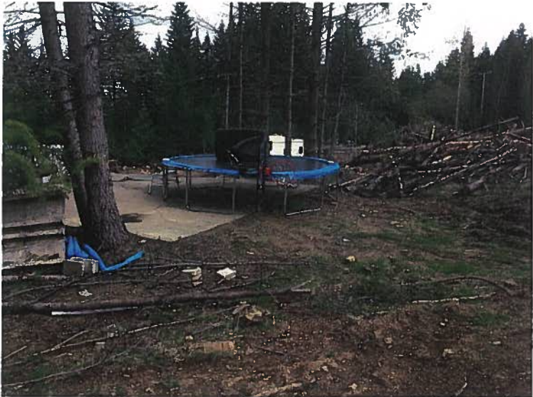
Figure 4 - Existing Concrete Pad
